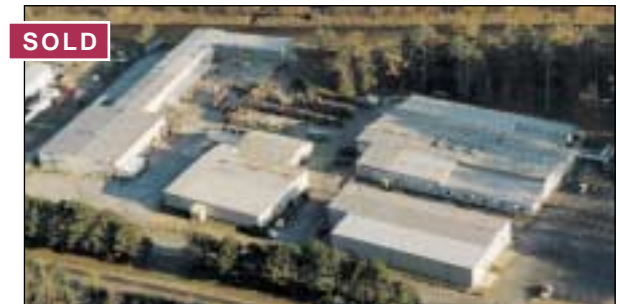
Former MacLean Power Systems: 106,453 sf. 14 acre site including 5 buildings totaling 106,453 sf. Purchased for future development. 6655 U.S. Hwy. 11, Trussville, AL. Agents: Jack Brown, sior & Ogden Deaton, sior Co-Agent: Howard Properties
