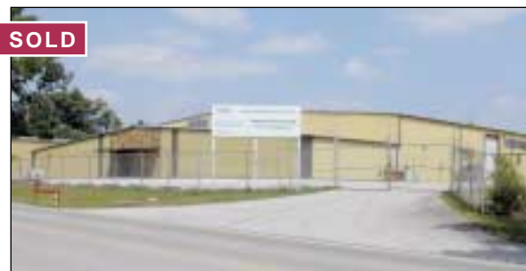
Former Buffalo Wire: 28,960 sf. Crane served manufacturing facility on 3.5 acres sold to Max Coatings. 3653 Industrial Parkway, Unincorporated Jefferson County. Agent: Jack Brown, sior • Co-Agent: Ogden Deaton, sior
