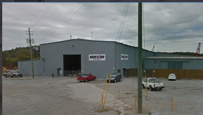
31,430 SF Industrial Building 2039 Fulton Springs Road, Alabaster, AL 12.1 Acre site
