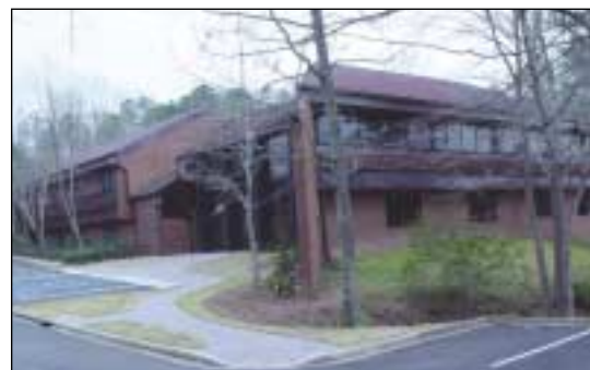
▲ - 501 RIVERCHASE PARKWAY - The law firm of Lamar, Miller, Norris, Haggard & Christie, PC relocated their offices to this recently renovated office on Chase Lake.
