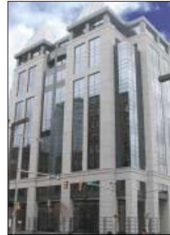
▲ - CONCORD CENTER - Birmingham's first new CBD Class-A office building in 12 years opened in March.
