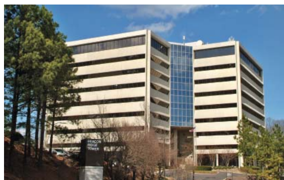
BEACON RIDGE TOWER Amsher Collection Services, Inc. renewed its lease of 16,964 sf in this Class A Vulcan/Oxmoor office tower.
